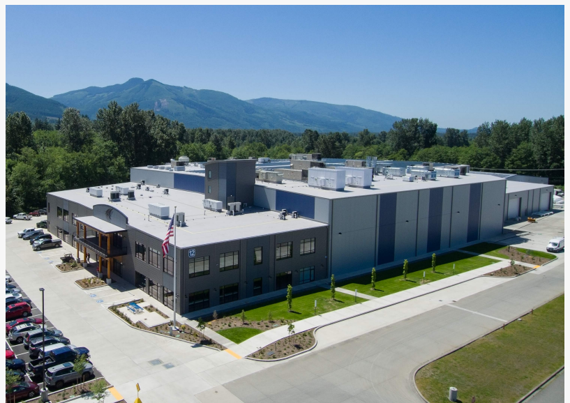
Janicki Industries Building 12 outside
