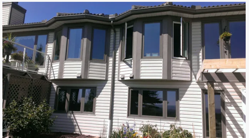
A completed project by the Window Seal West team.
