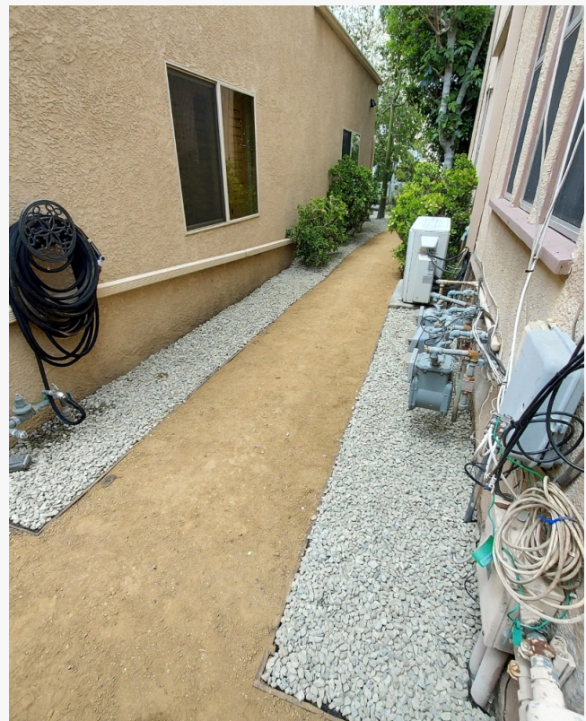
A commercial hardscape retrofit project featuring a decomposed granite walkway and gravel borders for effective drainage and erosion control.
