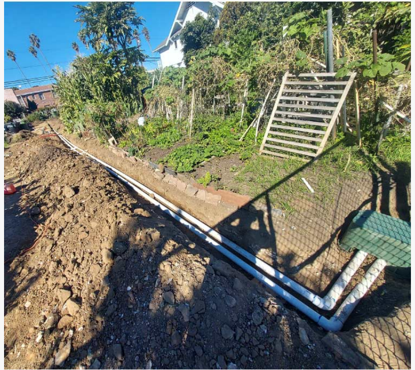
A newly installed commercial exterior side passage featuring decomposed granite walkways and gravel drainage borders to manage stormwater runoff.
