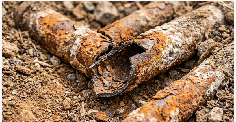
Aging cast iron sewer pipe, corroded and narrowed from decades of use.
