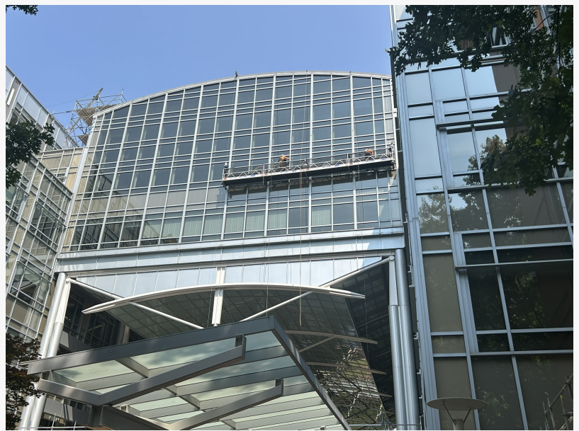
Western crews working on suspended scaffolding
