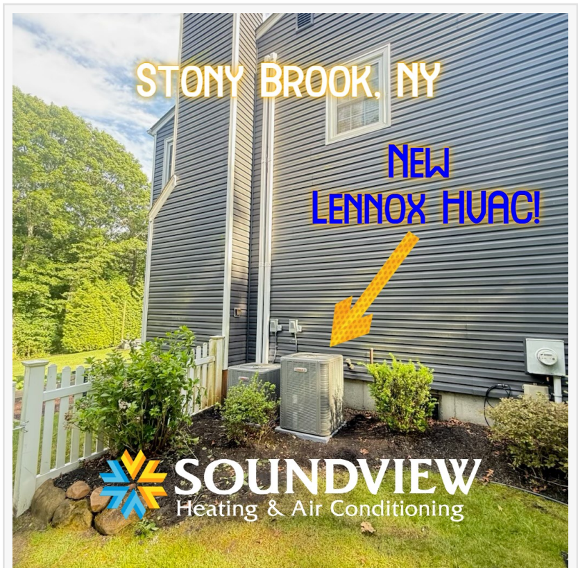
Lennox Heat Pump Installation in Stony Brook by Soundview HVAC
