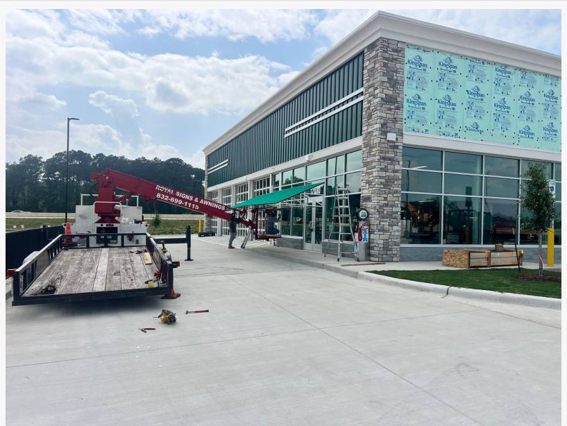
Royal Signs & Awnings at Mavis Tire site for installation
