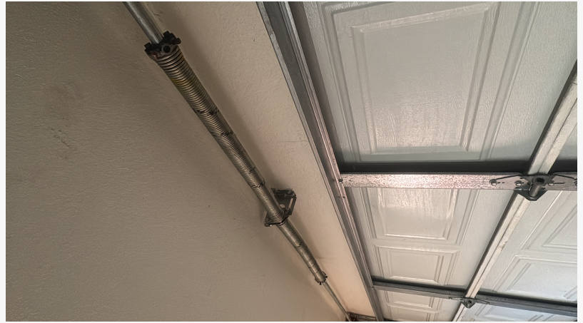
Emergency garage door spring replacement for broken springs in Long Beach, CA, provided by Garage Door Repair Long Beach By On The Spot.
