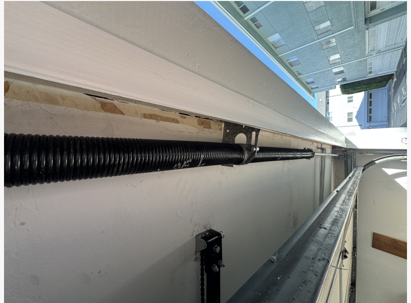
New garage door springs installed during a broken spring repair service in Long Beach, CA, by Garage Door Repair Long Beach By On The Spot.
