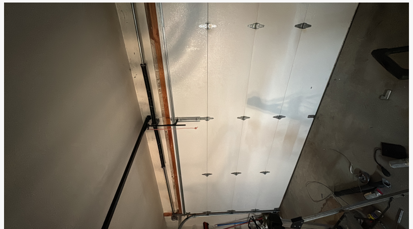
Late-hour emergency garage door spring repair in Long Beach, CA, helping homeowners restore safe and reliable garage door operation.
