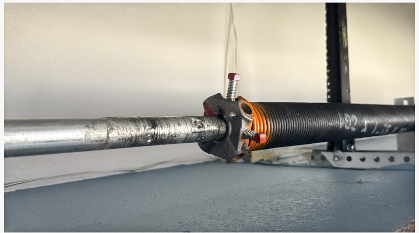
Affordable garage door tube and spring replacement in Long Beach, CA, helping restore smooth, safe, and reliable garage door operation.
