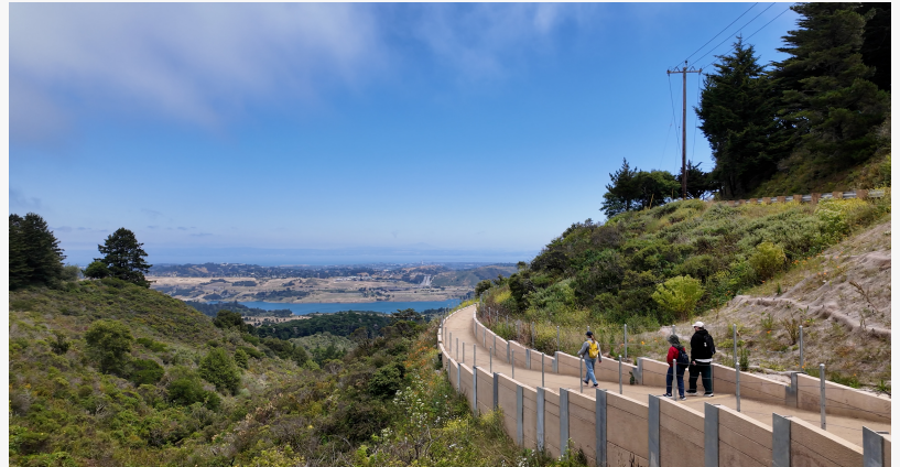
A bridge along the new six-mile Skyline Watershed Ridge Trail offers sweeping views.
