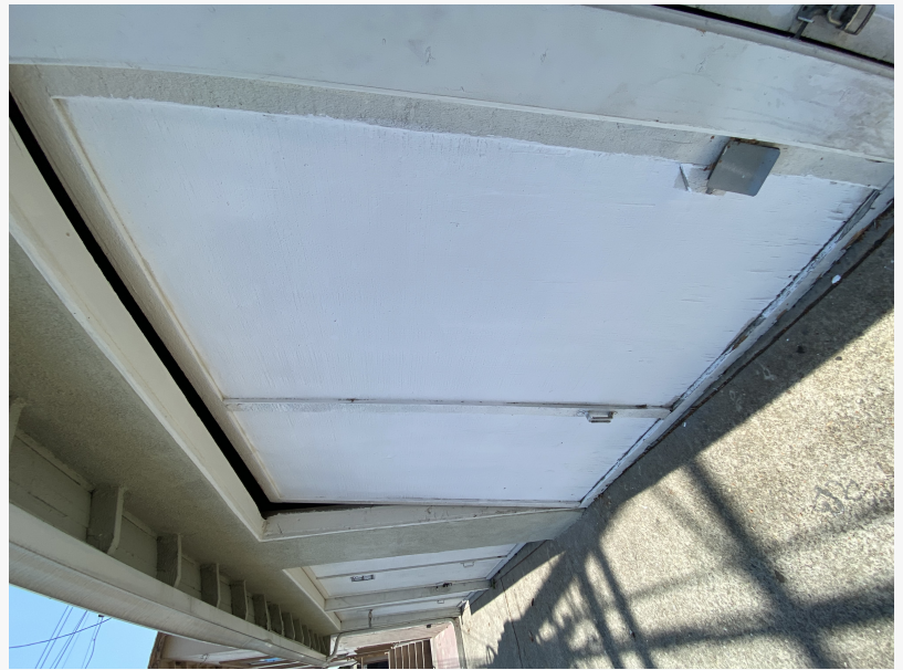
Emergency one-piece wood garage door repair in Santa Clarita, CA, provided by Next Hour Garage Door Repair Santa Clarita.
