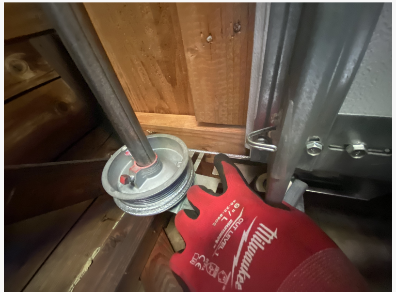
Emergency garage door cable replacement in Stevenson Ranch, CA, helping restore safe and reliable garage door operation.
