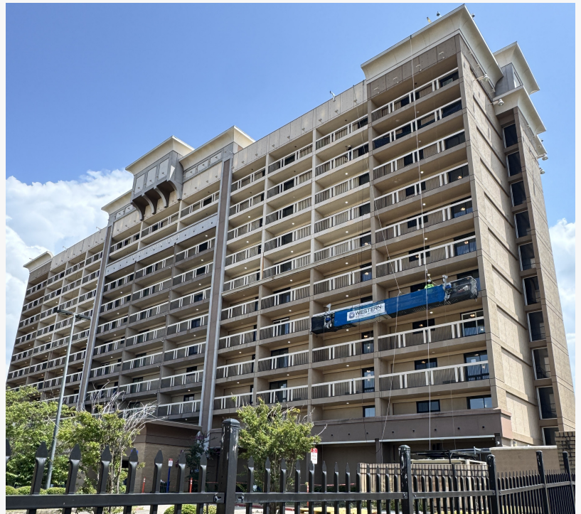
Western's swing stage on Venson Towers
