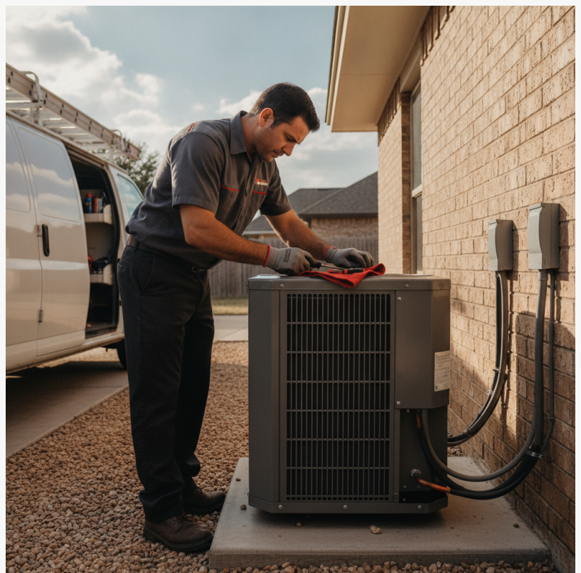
A Mission Air Conditioning technician repairs an outdoor AC unit in McAllen, TX, where emergency service calls spike each summer as temperatures push past 100°F.
