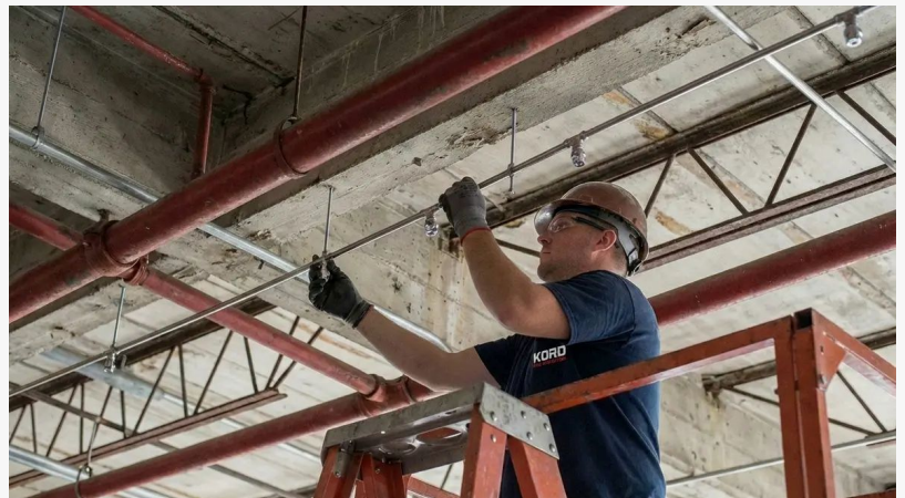
Fire Sprinkler Work
