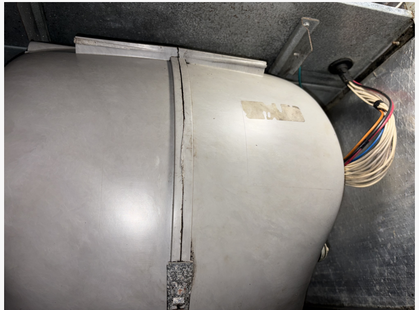
Air Duct Cleaning After
