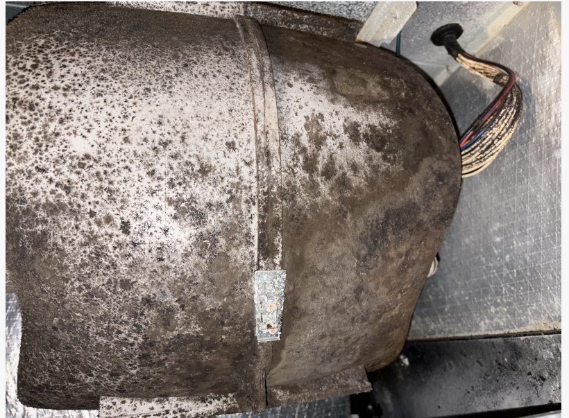
Air Duct Cleaning Before
