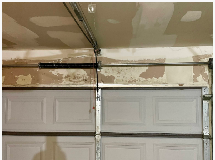
Garage door spring replacement service in Houston, TX, helping restore safe, balanced, and reliable garage door operation.
