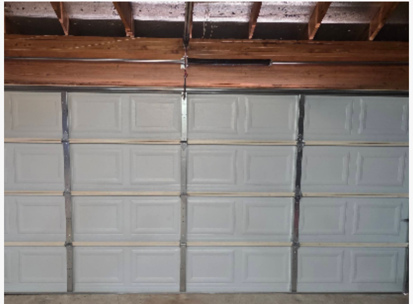
Garage door spring repair service in Houston, TX, helping restore safe, balanced, and reliable garage door operation.
