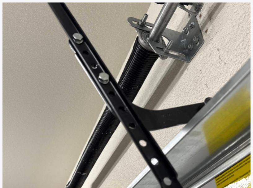
Garage door torsion spring replacement in Las Vegas, NV, helping restore proper balance, safe lifting, and reliable garage door operation.
