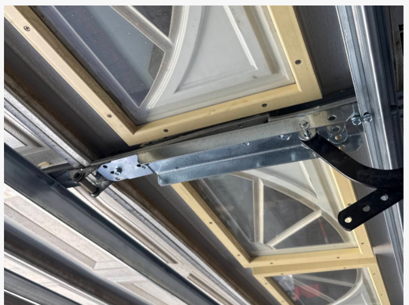
Garage door reinforcement strut and opener bracket repair in Las Vegas, NV, helping strengthen the door and support reliable opener operation.
