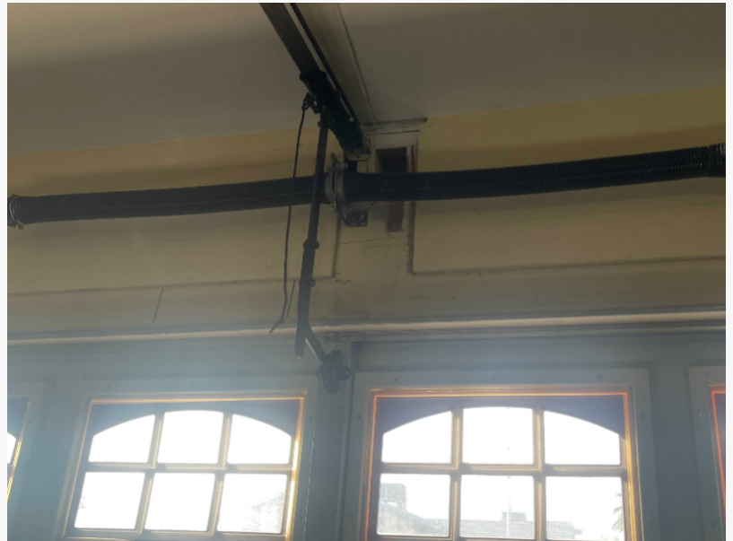
Garage door strut bar replacement in Las Vegas, NV, helping reinforce the door panel and support safe, reliable garage door operation.
