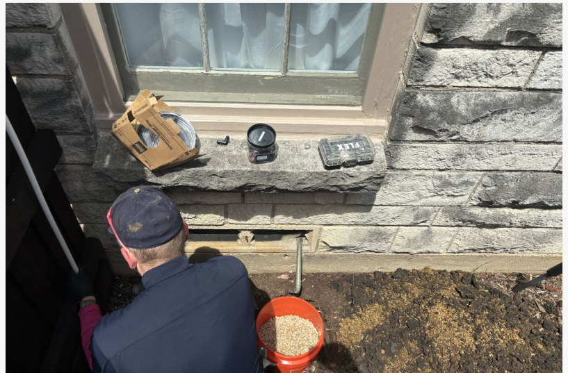
A Mother technician repairs a residential gas line in Dallas.
