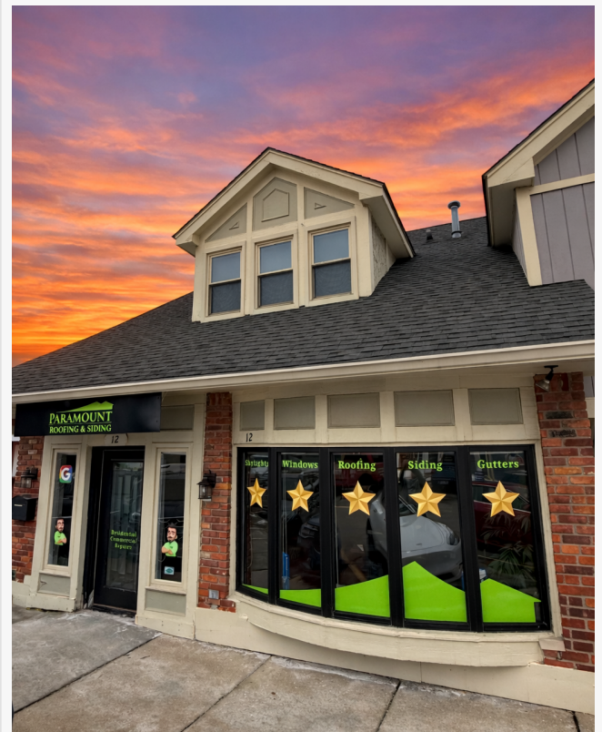
Paramount Roofing - Plymouth Location
