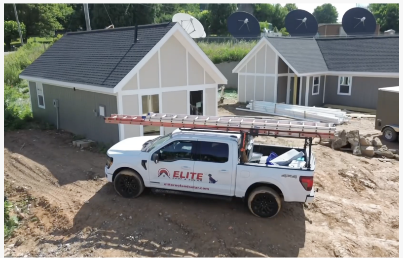
Sawmill Village's Fortified Roof Installation by Elite Roof and Solar
