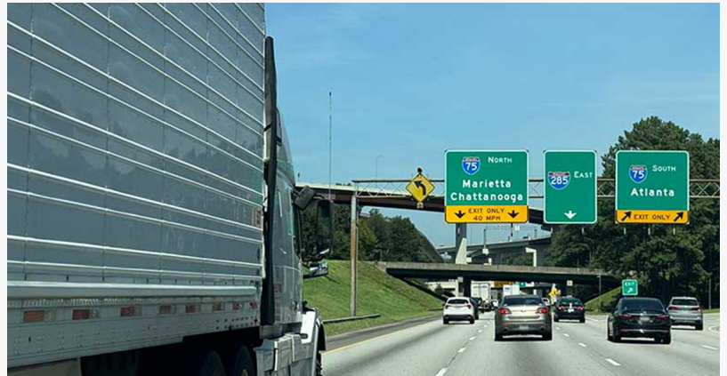
dangerous roads and intersections cobb county ga
