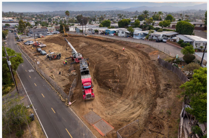
Aerial view of the Caritas Village – Vista site following initial site preparation in Vista, California. Level 3 Construction has begun early construction activities for the 24-unit affordable housing community being developed by The Caritas Corporation.
