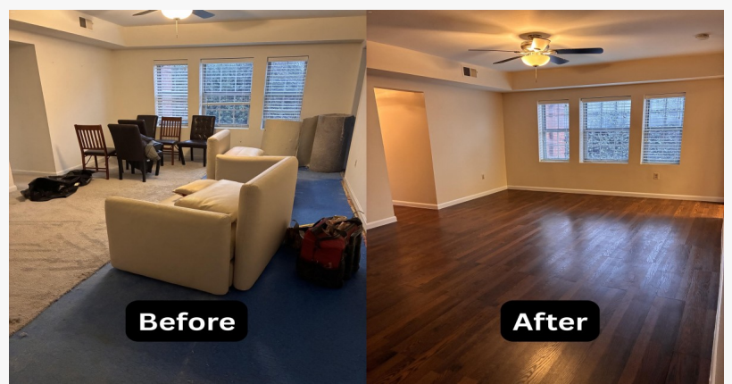
Before and after: Eagle Eye Construction transformed this Rosslyn, Virginia apartment with new LVP flooring and a full interior repaint.
