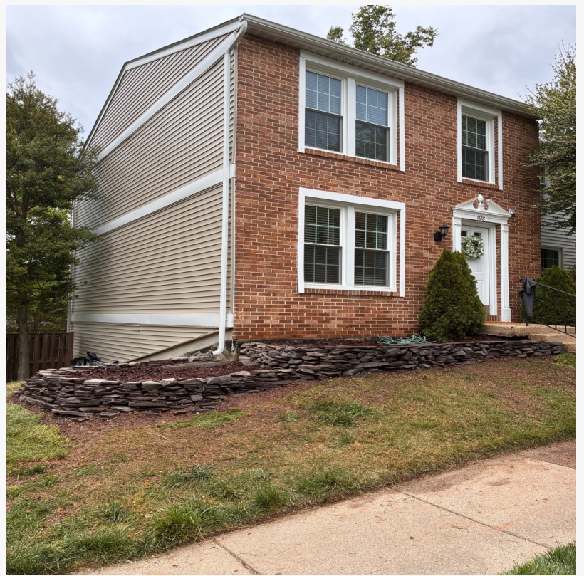
A completed natural stone retaining wall and drainage project by Eagle Eye Construction in Reston, Virginia.
