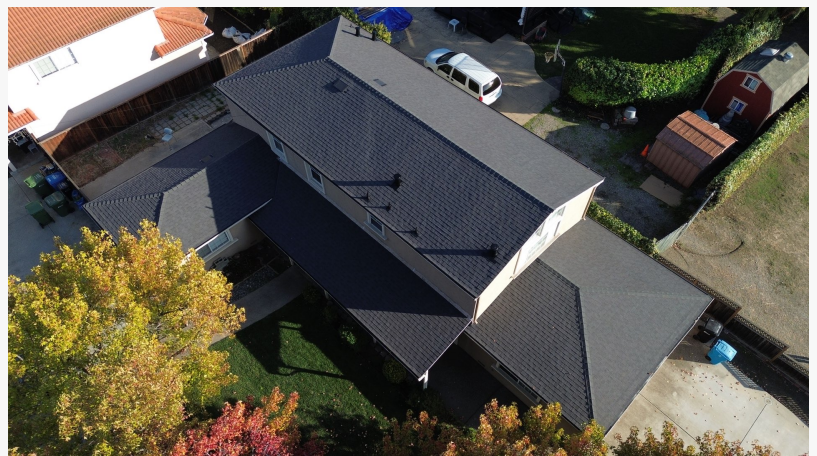
Completed roofing project in san jose ca
