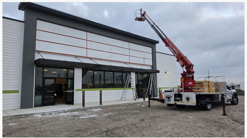
At Refuel site, during installation
