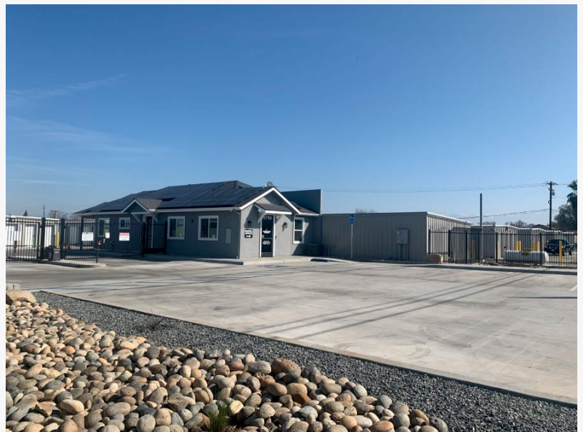
Front office and secure keypad access entrance at Freedom Storage Inc. in Visalia, CA.
