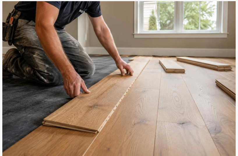
Engineered hardwood flooring installation in Moncks Corner SC
