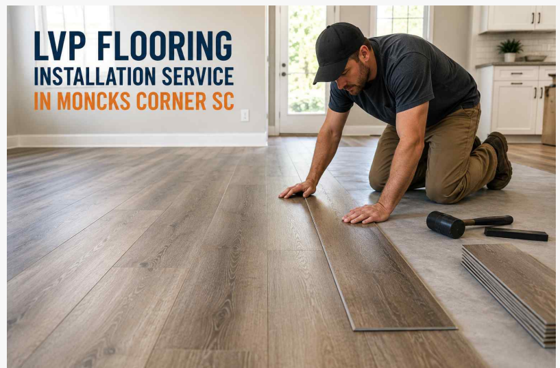
lvp flooring installation service
