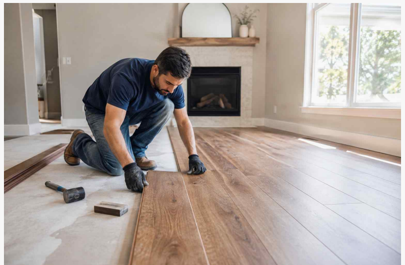
flooring installation for homeowners
