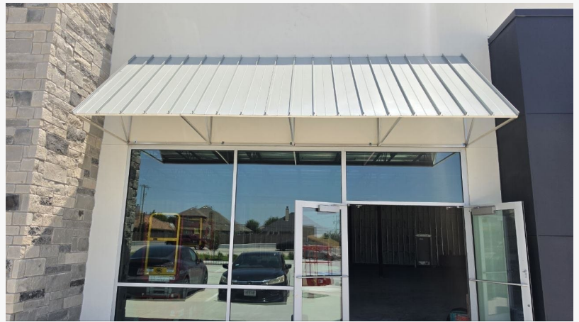
Standing Seam Awning for Victory Forney East
