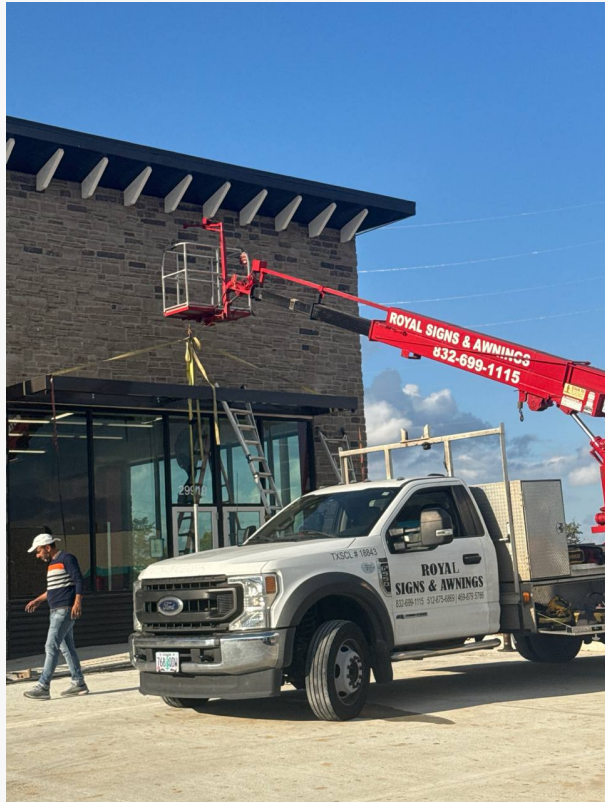
Installation in-process at AutoZone
