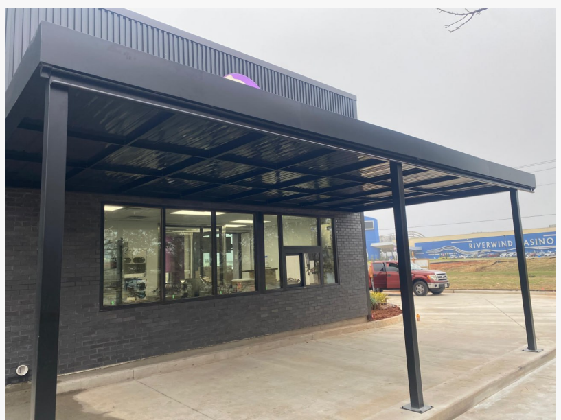
Metal Canopy installed for Taco Bell
