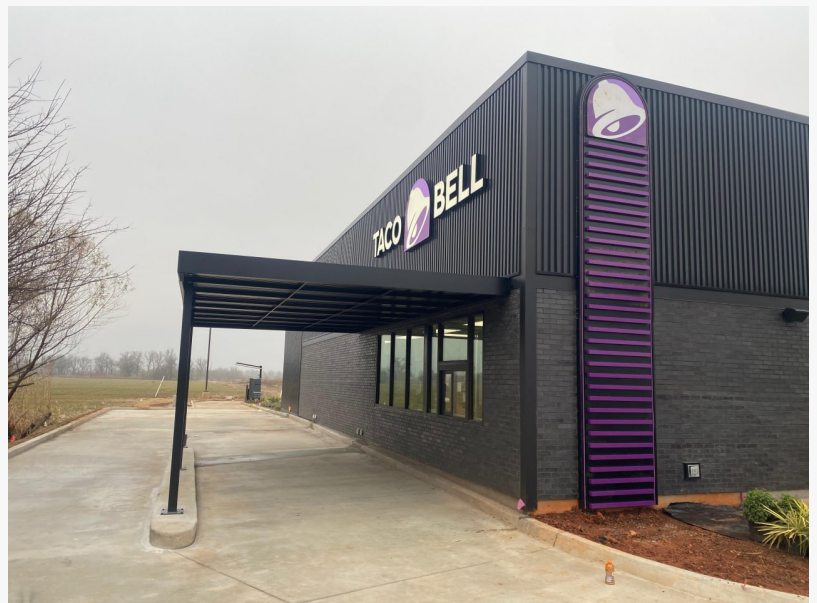
Canopy installation for Taco Bell- New Castle
