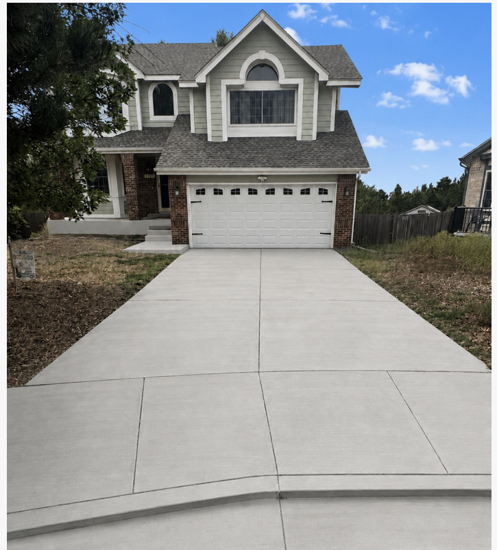
Concrete Driveway Replacement in Colorado Springs
