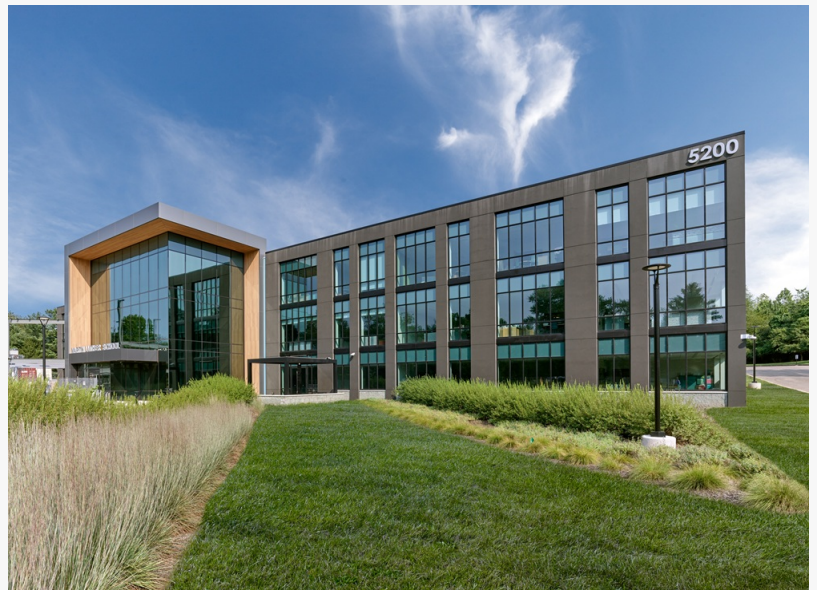
Phase I construction on Martin Luther School, an innovative educational environment in the Philadelphia region, has been completed.
