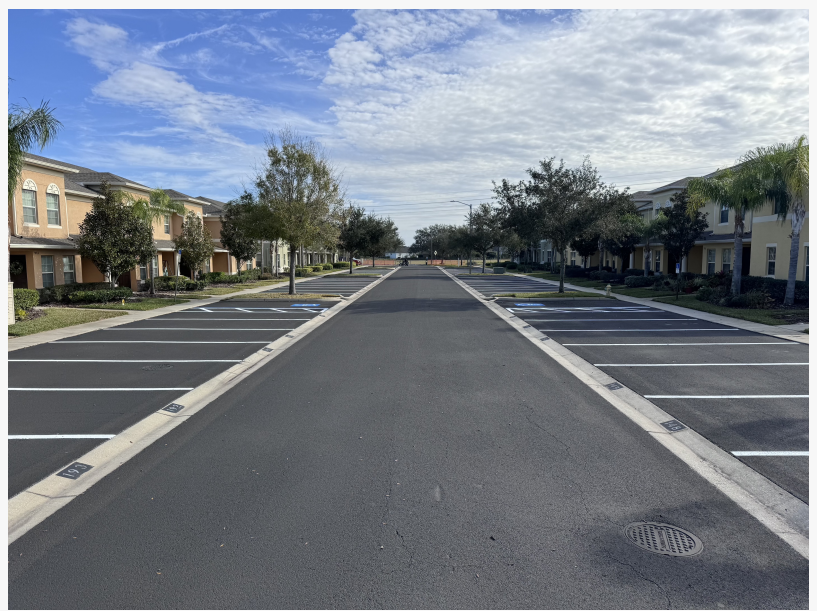
Paving the Way: Express Asphalt Solutions Brings Premier Asphalt Services to Orlando's Growing Infrastructure Needs
