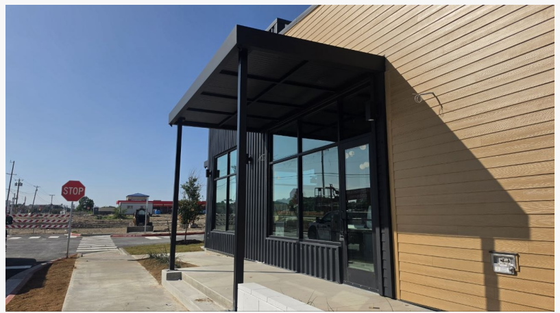
Metal Canopies installed for Black Rock Coffee
