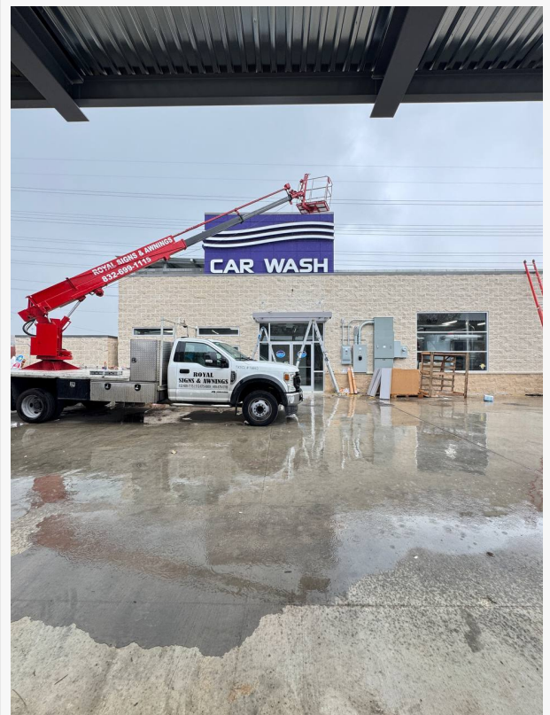
Installation process at White Water Express Car Wash
