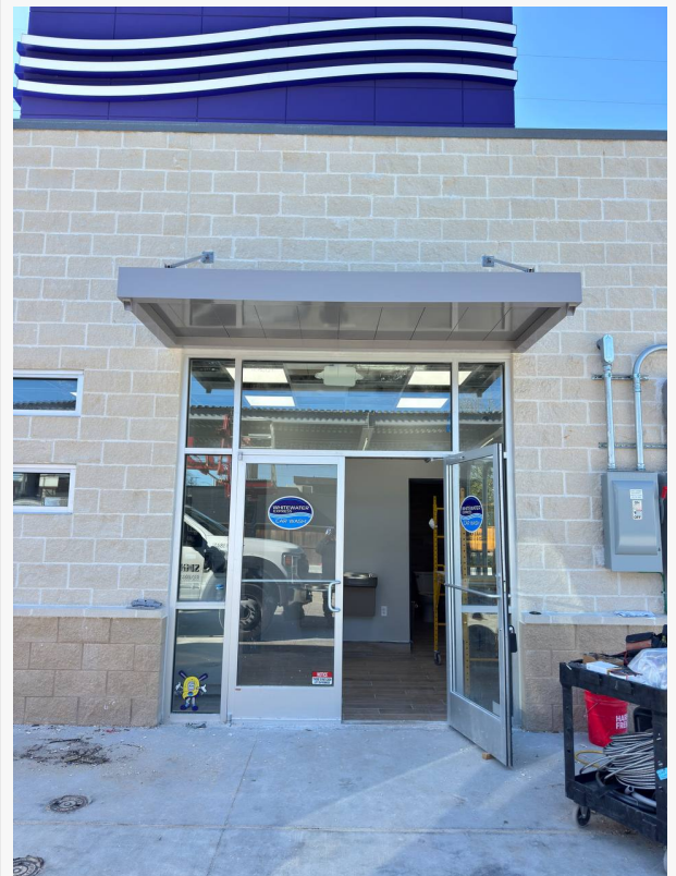
Installation completed for White Water Express Car Wash
