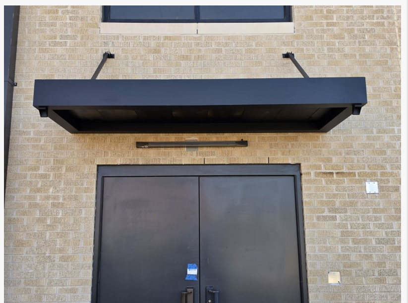
Metal Canopy installed for Austin Elementary School
