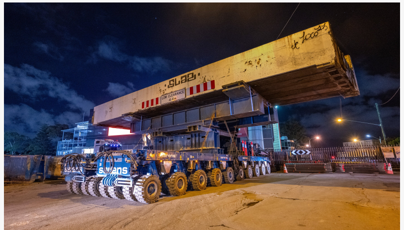
Sarens deploys Crane+ model in Australia
