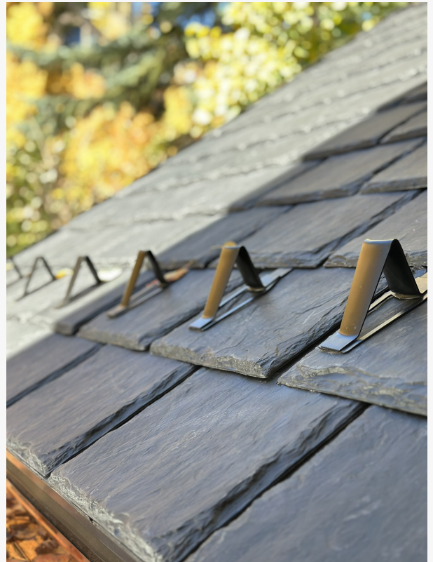
Powder-coated Everest 16 snow guards placed on a DaVinci Slate roof require no maintenance and will help keep snow from avalanching off the synthetic roof.
