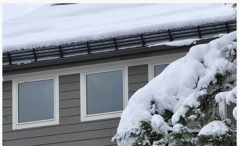
Drift Solar Snow Fence from Rocky Mountain Snow Guards helps snow that has slidden off a solar panel stay on the roof, so it can melt slowly and safely.
