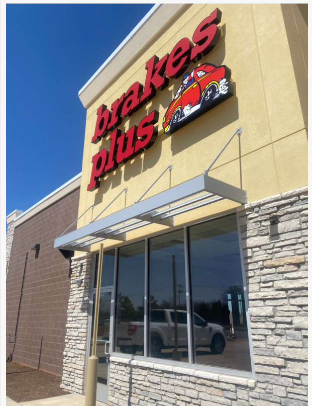
Metal Canopies installed for Brakes Plus
