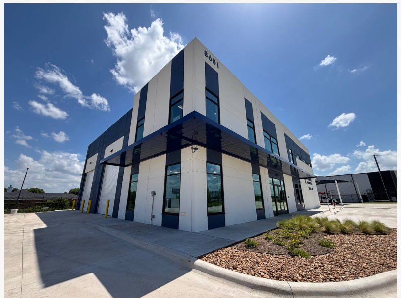
Metal Canopies Installed for SDF Dental Hub
