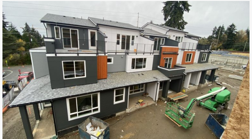
Siding Contractor | EvoSiding Vancouver WA
