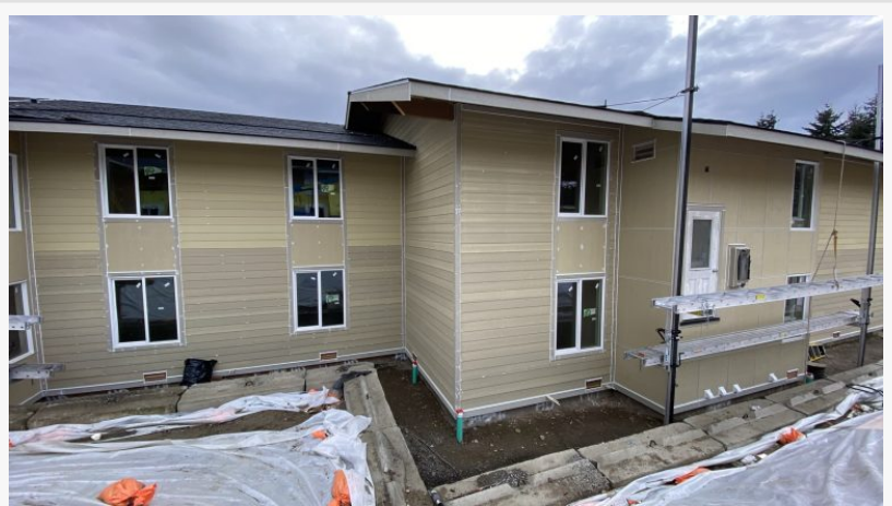
Siding Repair | EvoSiding Vancouver WA
