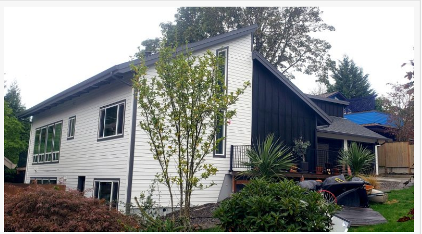
Siding Replacement I Vancouver WA
