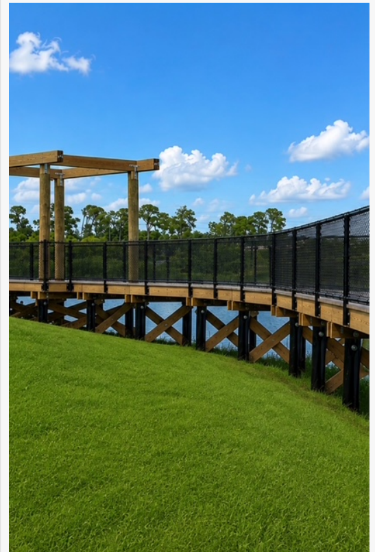
Boardwalk at Crystal Lake Fence
