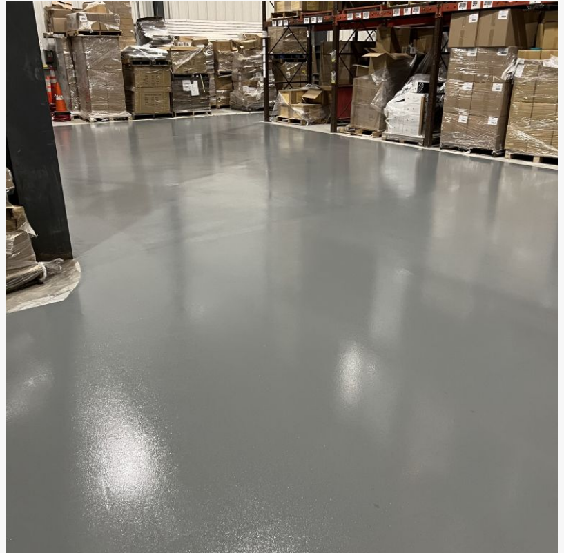
WAREHOUSE EPOXY FLOORING
