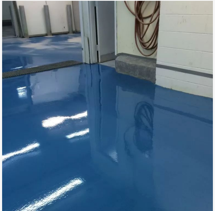
Epoxy Flooring Tri-State Contractor
