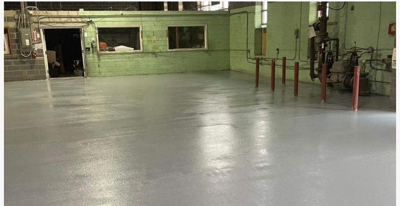
Warehouse Epoxy Flooring
