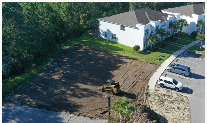
Site work underway at Hidden Forest in August 2026 — grading for the Hidden Forest Clubhouse beside the existing townhomes.
