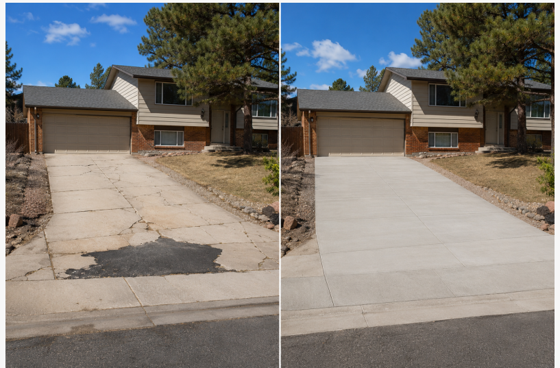
Concrete Driveway Replacement in Colorado Springs 5
