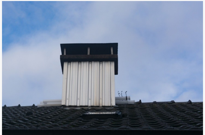
chimney repointing services in Stayton, OR
