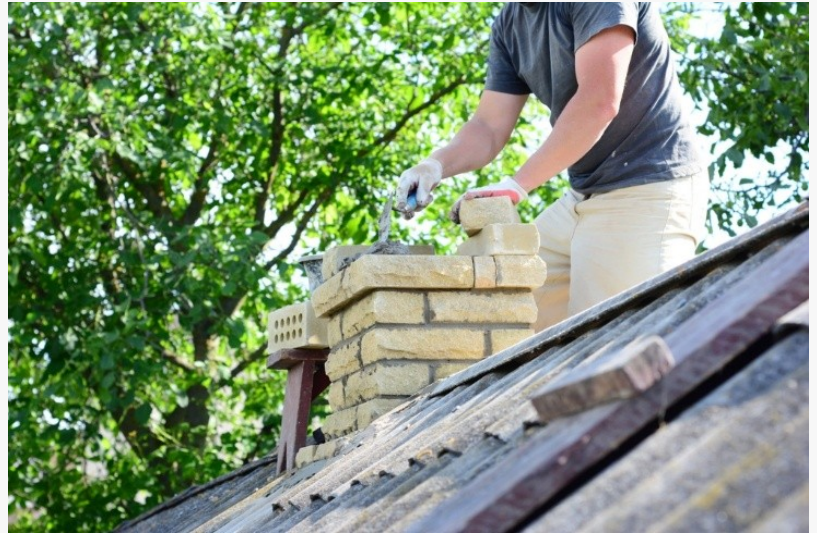
chimney brick repair in Stayton, OR
