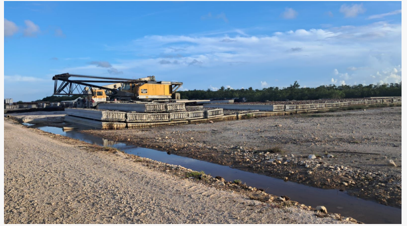
Construction begins at Olo Caye's mainland facility in Belize City.
