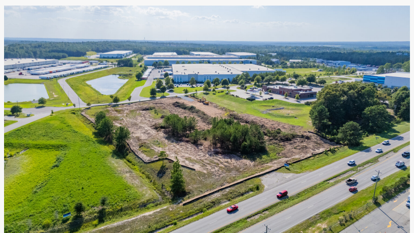
BEHKO Construction & Magnus Development Partners break ground
