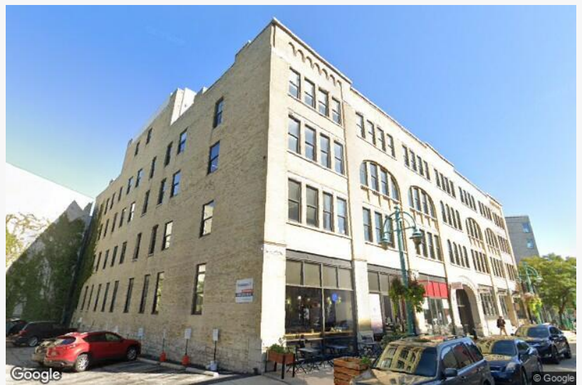
222 E. Erie Street owned by 222 Property Owners, LLC
