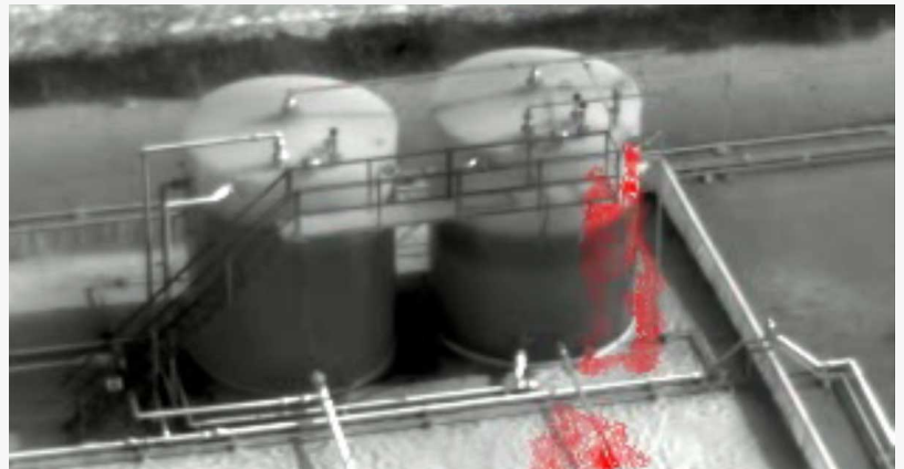
PAM detects gas at a tank farm
